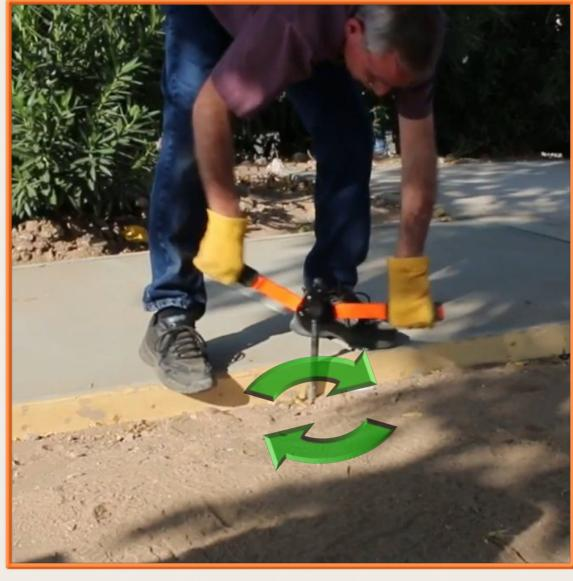
While firmly gripping the stake, rotate the stake by using a twisting motion to break the surface tension.
